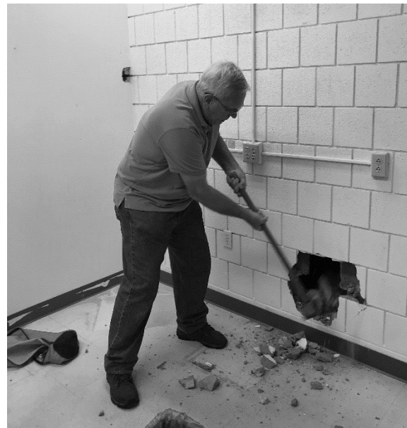
Dean begins the renovation
