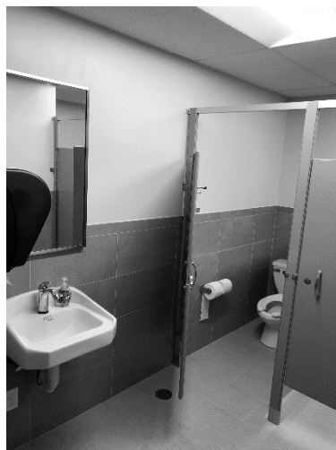
Women's room- completed
